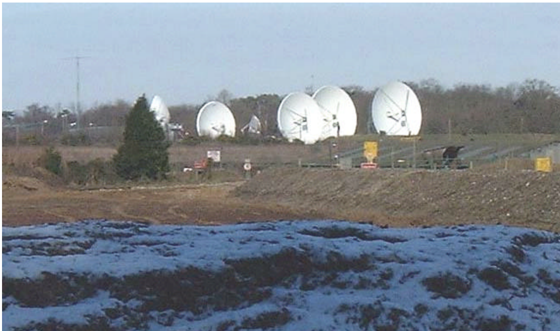
Dishes at BT Adastral Park Earth Station
