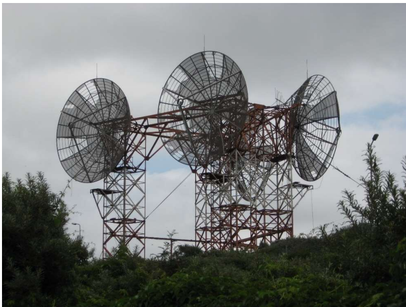
Photo of Hoek van Holland tropo scatter station that is no longer in use
