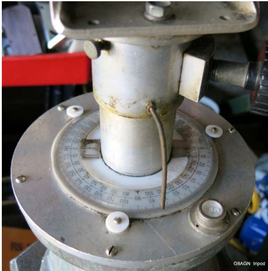
Figure 3 Dish mounting showing rotatable protractor
