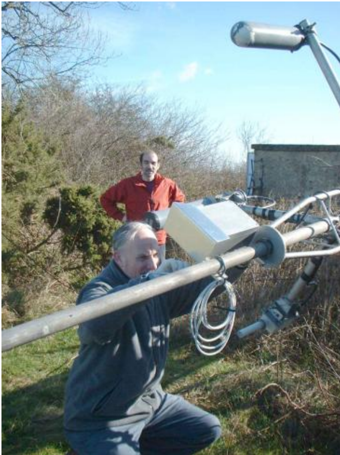
Chris G8BKE tightens the U bolts holding the beacon assembly observed by Andy G4JNT.
