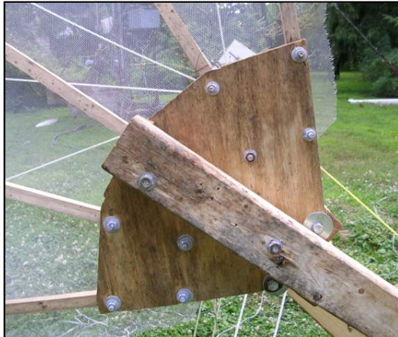
Figure 5: Spokes are attached to a plywood center hub with two bolts each.
