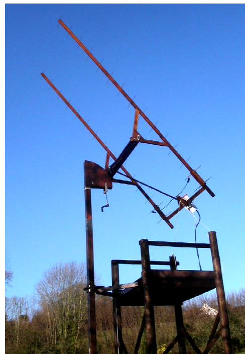
Figure 6: Antennas on East tower
